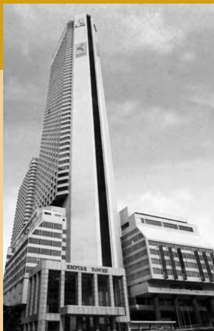
The 3-in-1 integrated commercial complex known as City~Square Centre comprising the Empire Tower, City~Square Shopping Centre and Crown Princess Kuala Lumpur.
