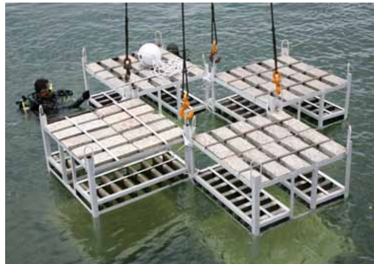
Artificial ceramic corals invented by SIRIM help natural coral habitats to regenerate.
