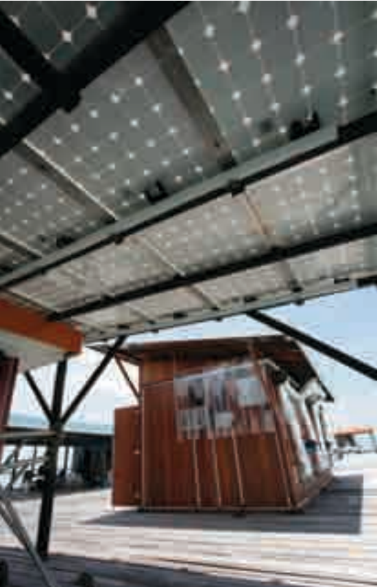
Solar-powered seaweed dryer system in Sabah
